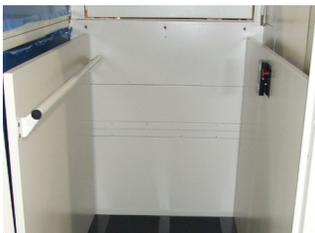
Straight through car with paddle controls and hand rail
