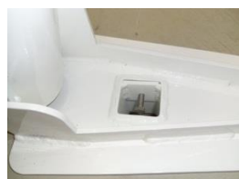
3/8" bolt inside anchor sleeve
