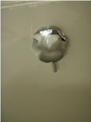
← Shown Here is Overflow & Drain Knob
